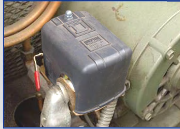
Air Pressure Switch
